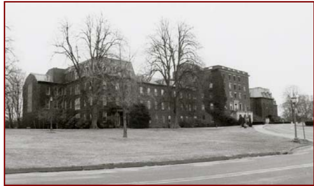
Connecticut Valley Hospital
