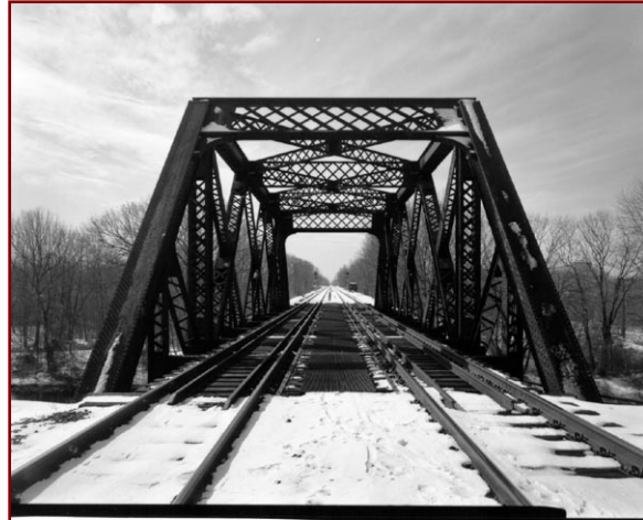
Pawtuxet River Bridge, Cranston, RI
