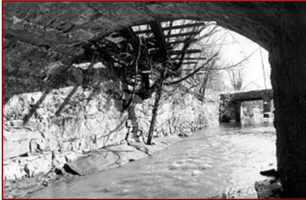
Millbrook Sewer Portal, Worcester, MA
