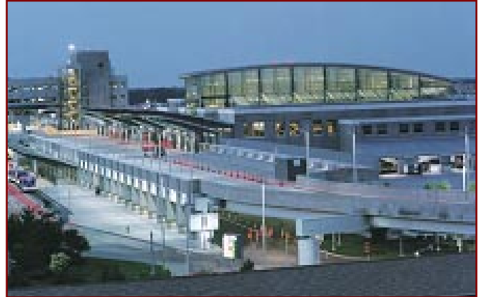
T. F. Green Airport Main Terminal
