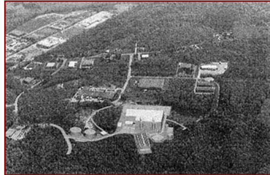
Aerial Photograph of the AES Londonderry Cogeneration Facility
